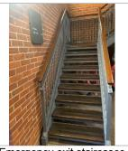
Emergency exit staircases Staircase: 88cm W / steps: 18cm H / 1 x handrail.
